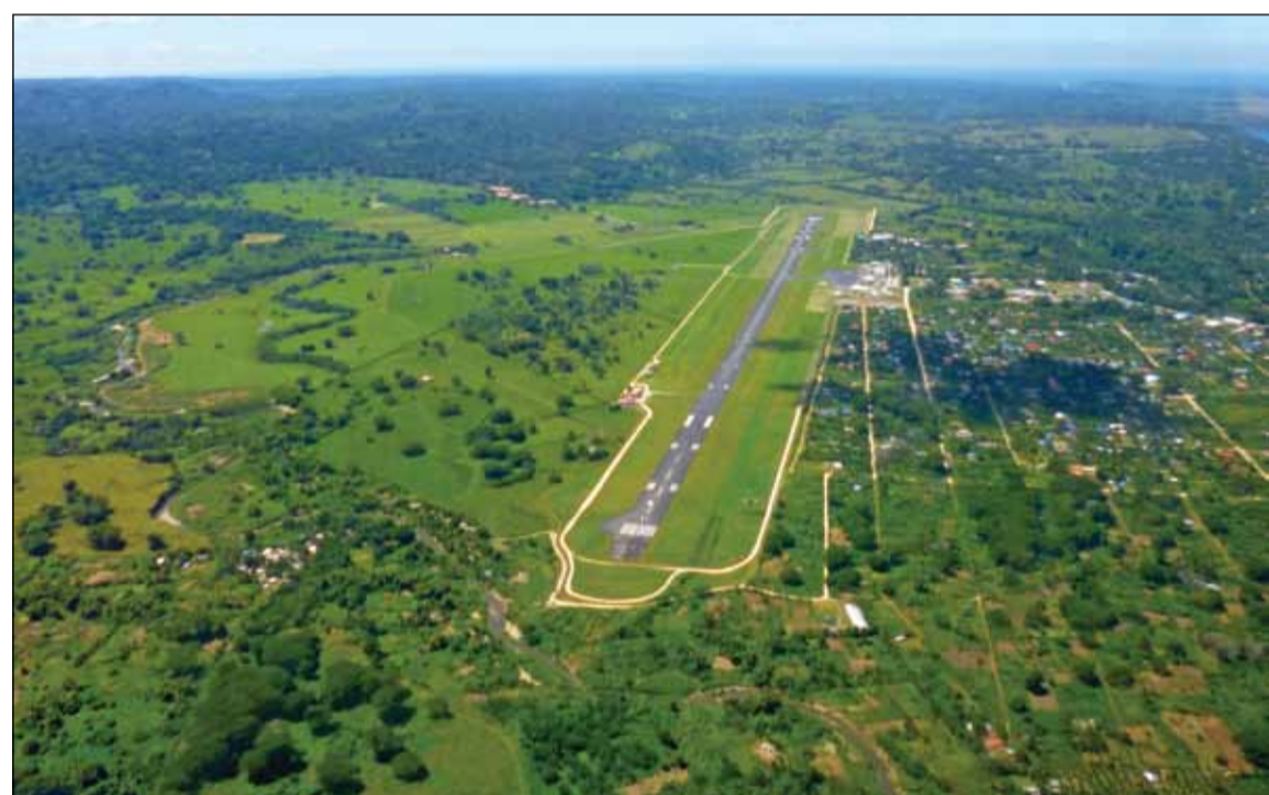
The international airport at Port Vila is receiving an upgrade.
