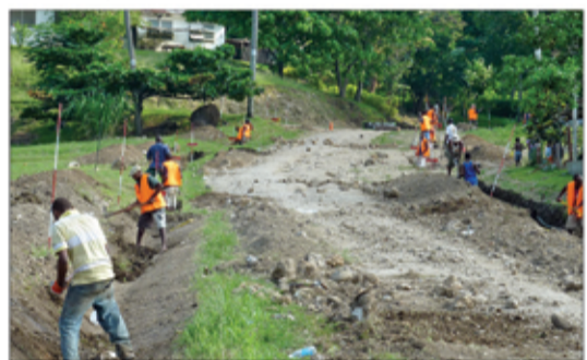
Building the roads to improve life for all
