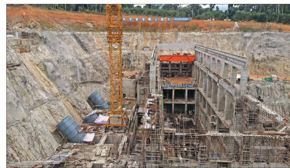
Work on the Memve'ele Hydro-power Dam is ahead of schedule.
