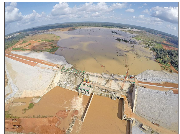
The Lom Pangar dam maximizing Cameroon's hydropower potential.
